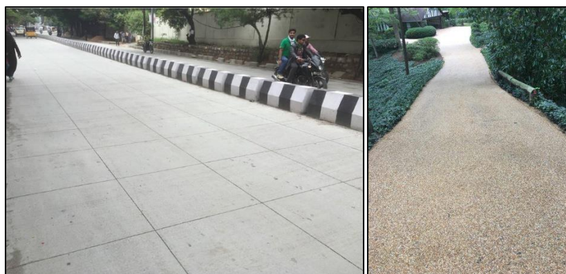
Figure 103: Example of whitetopping (left) road design, as well as applied chip seals with light-colored aggregates. Source: Intra Construction & Equipment Magazine, https://bit.ly/3hhw9Cj (12.03.2021).
