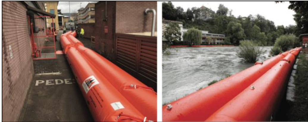
Figure 92: Example of hose dam embankment systems. Protection of water along rivers and exposed residential buildings. Source: https://www.xh020.com (02.03.2021).
