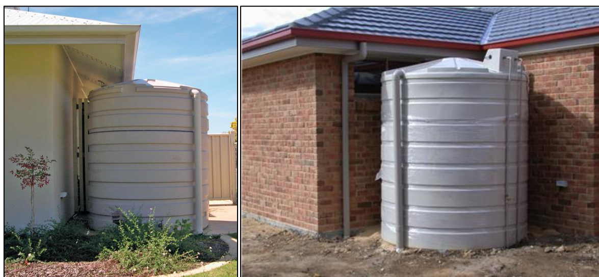
Figure 91: Example of water collection tanks for buildings (e.g. residential buildings or public buildings). Source: https://www.rainfilltanks.com.au (26.03.2021).
