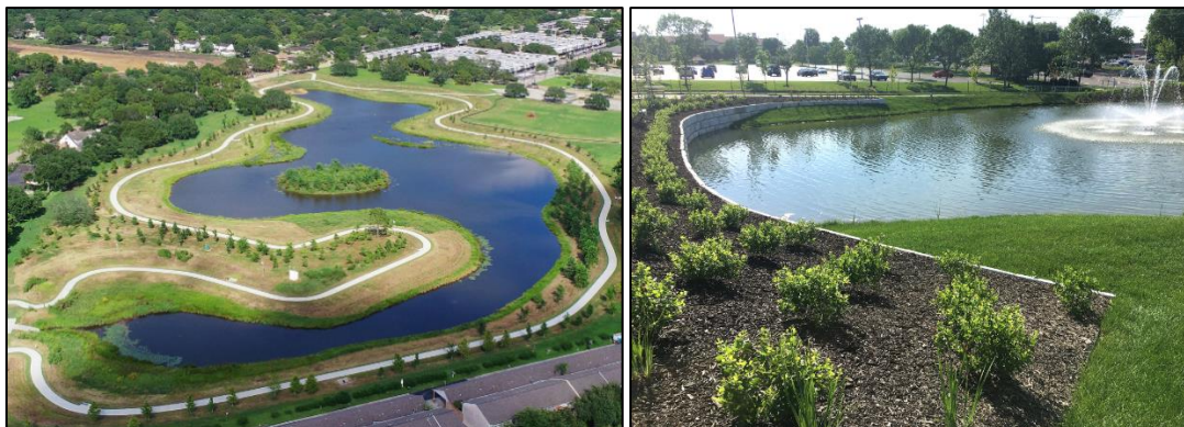
Figure 83: Examples of retention reservoirs/ponds. Source: https://bit.ly/3ojiMaw (17.02.2021).
