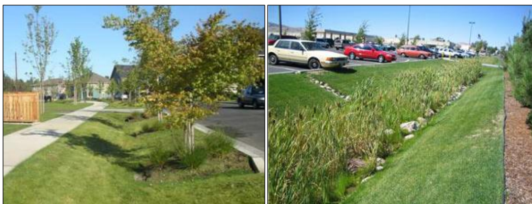
Figure 84: Examples of vegetated swales along roads and parking areas. Source: https://dottarchitecture.com (18.02.2021).
