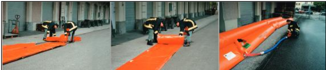
Figure 93: Example of the installation process of the hose dam segments. Lay out and position, inflate with air and fill with water. Source: https://www.flexdamm.de/docs/Beaver-Prospekt2016.pdf (02.03.2021).
