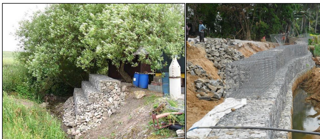
Figure 39: Example of installed gabions to restore and stabilize riverbanks.
