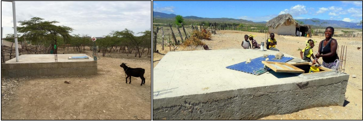
Figure 40: Examples of cisterns made of reinforced concrete.
